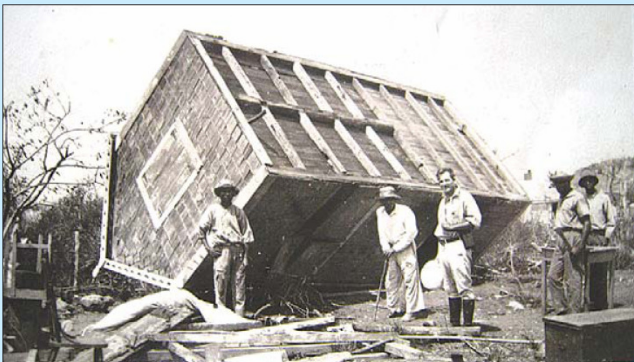
Mr. Lampe remembers his first hurricane, in 1924. He was not impressed, and still is not: "Simply hook up your house," something the owners of this house obviously failed to do in 1924. (One of Lampe's many photos documenting the past).
